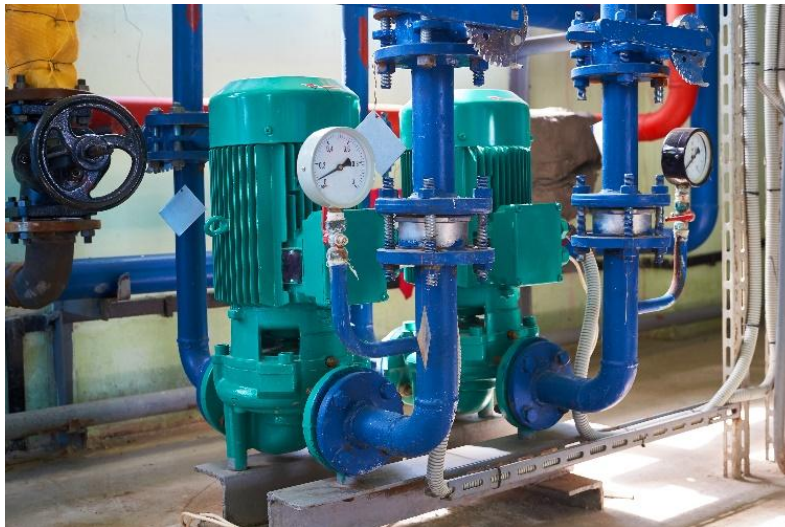
Figure 3: Pump with a three phase electric motor
