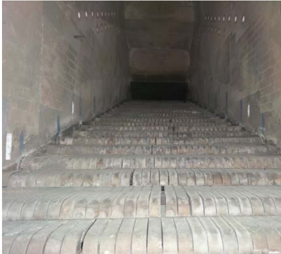
Figure 11: Boiler Grate Internal View
